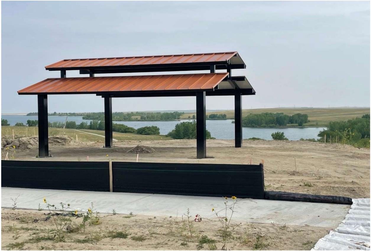
Filing 17 Gabled Shade Structure at Overlook Park
