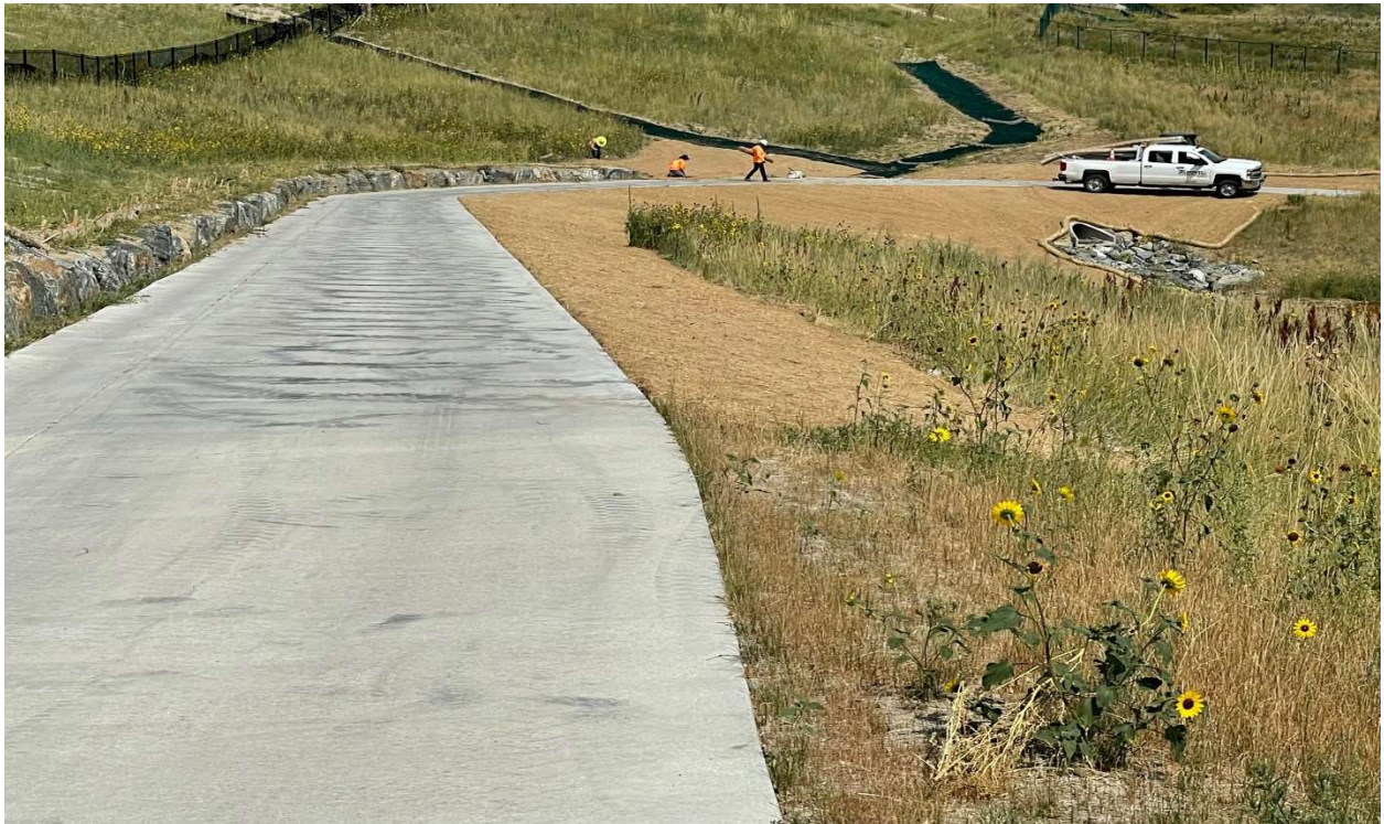
Grading and erosion control work around Pond C
